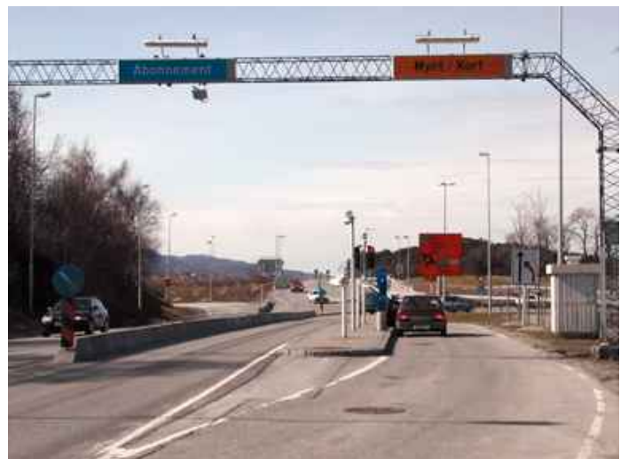
Automatic toll plaza in Trondheim
