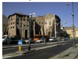
Access control gate in Rome city centre
